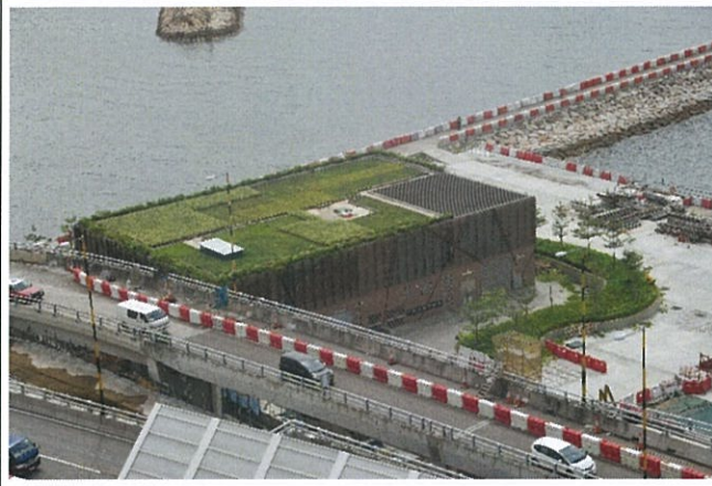
V1 - East Ventilation Building
