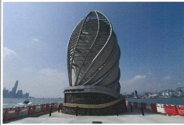
V7 – East Ventilation Shaft
