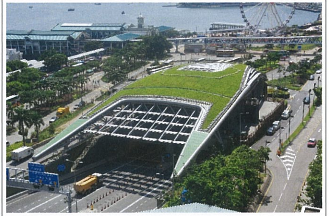
V2 – West Ventilation Building
