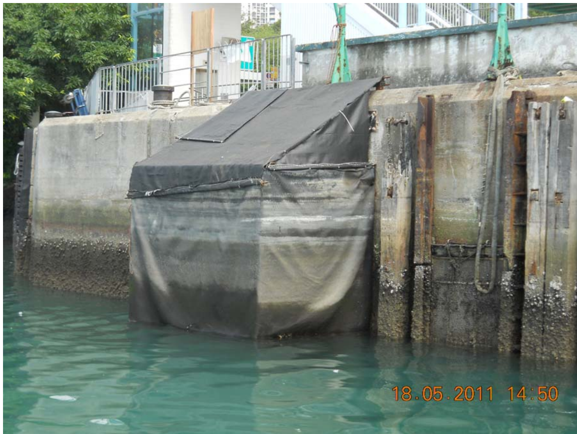
Installation of silt screen at cooling water intake (Windsor House)
