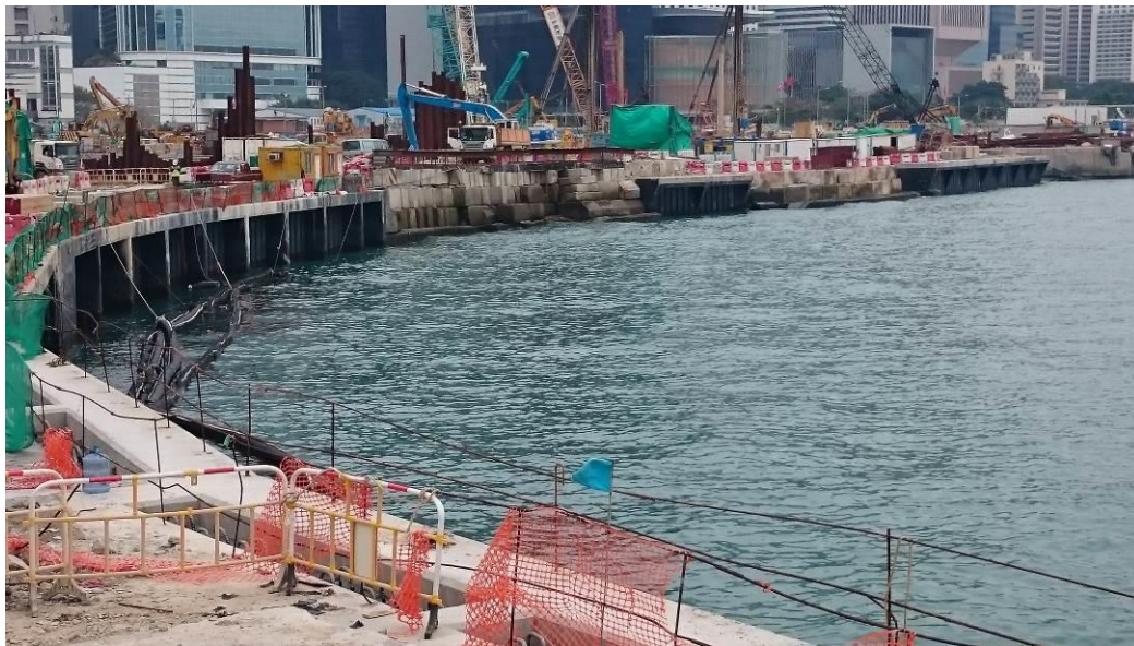
Site towards the West on 19 Dec 2015
